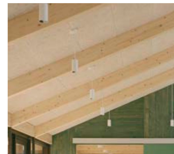
Interior - Simple plywood finishes with exposed beams
