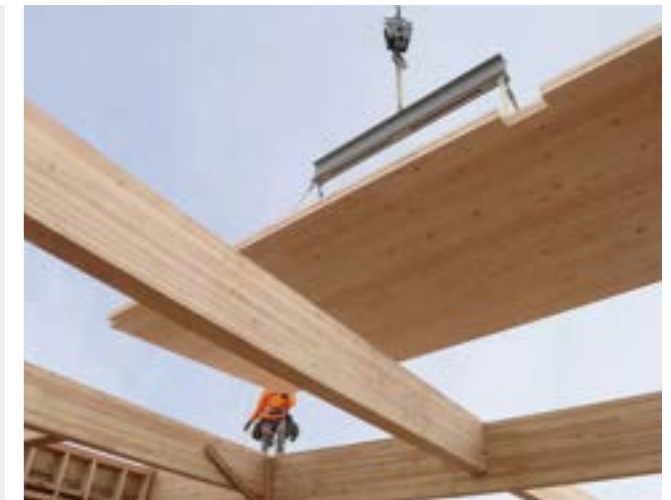
Off-site prefabrication
