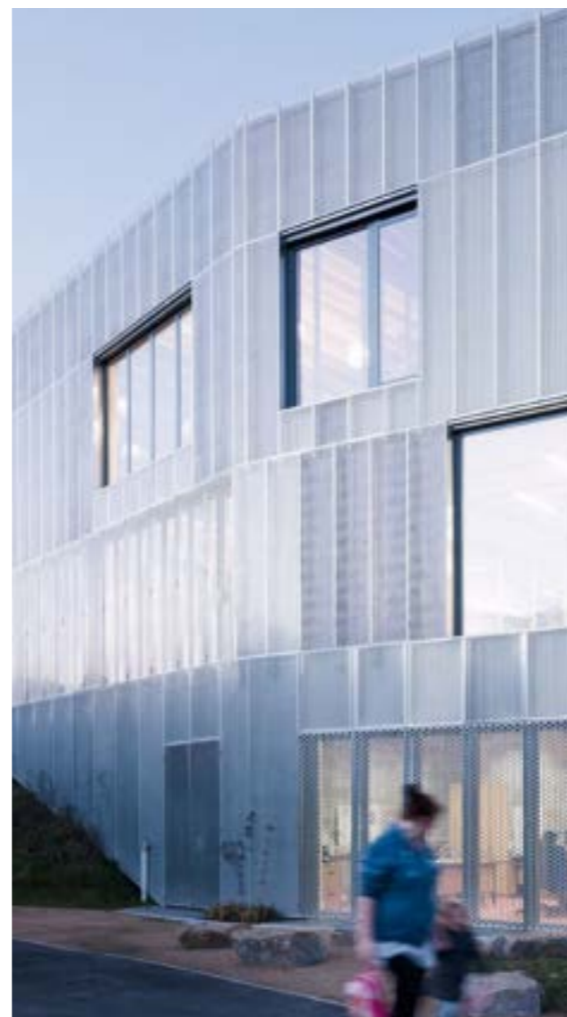
Cladding - perforated profiled PPC metal. Profile tbc
