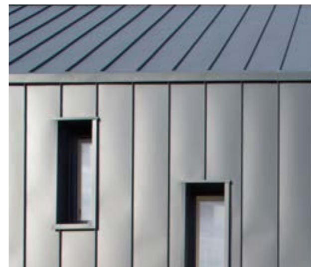
Roof & Canopy - preformed standing seam steel
