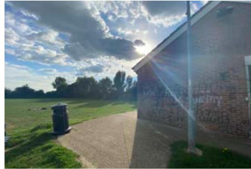
1. South view looking past Knoll Pavillion, towards recreational ground
